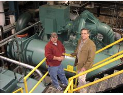
Bruce Stultz (right) with Central Plant Manager Mike Penyak and a new chiller in a DGS facility.
